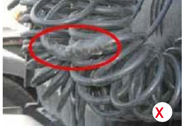
Running lines and cables.
