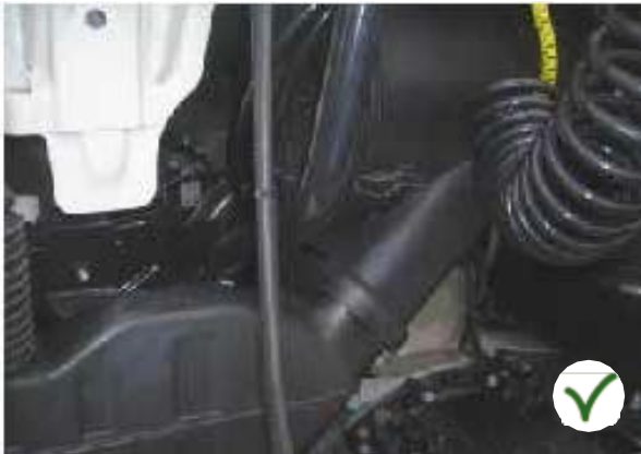
Air intake housing
