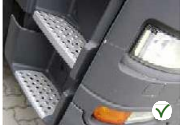
Entry normal wear and tear.
