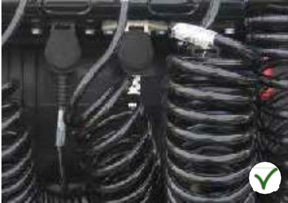
Running lines and cables.
